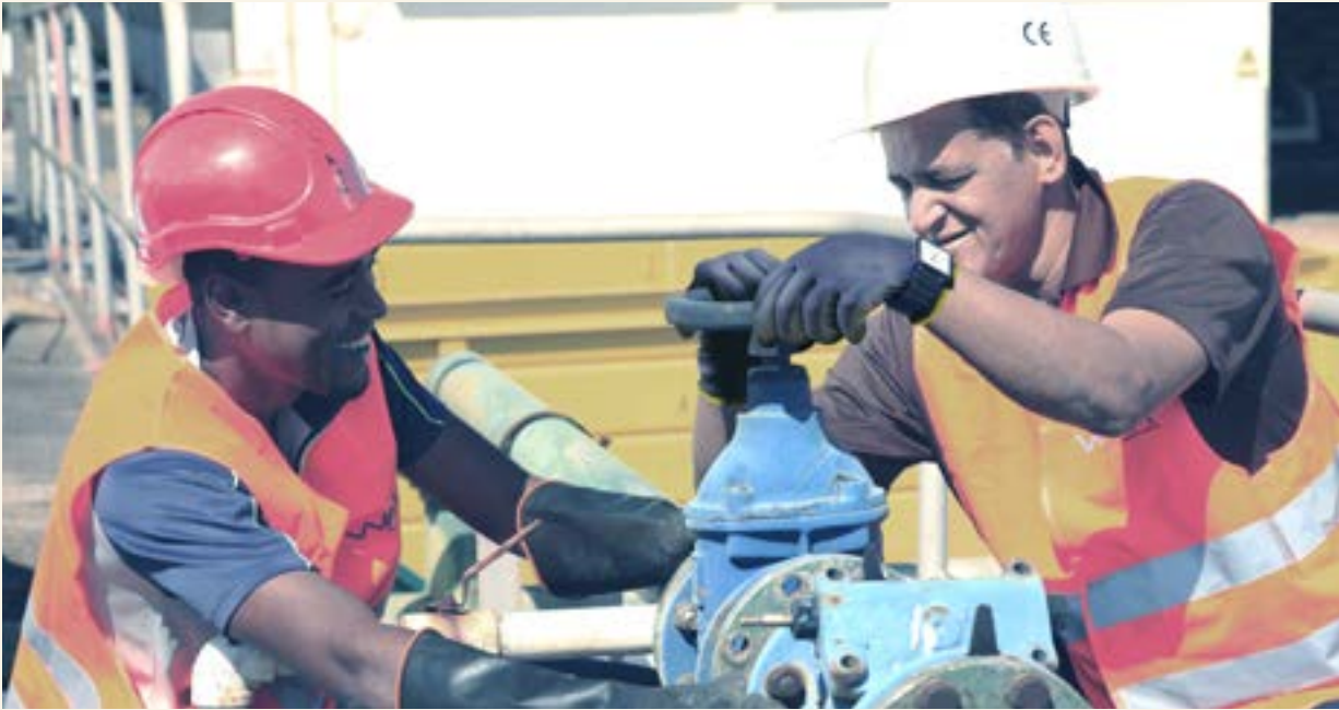
Maintenance on gate valve
