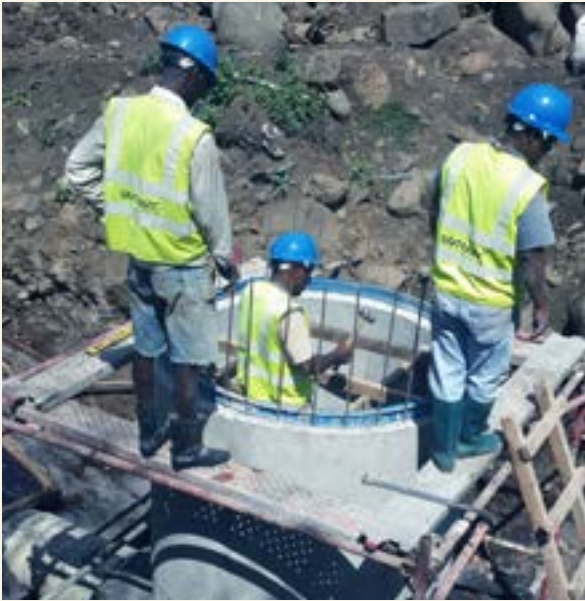
Manhole construction
