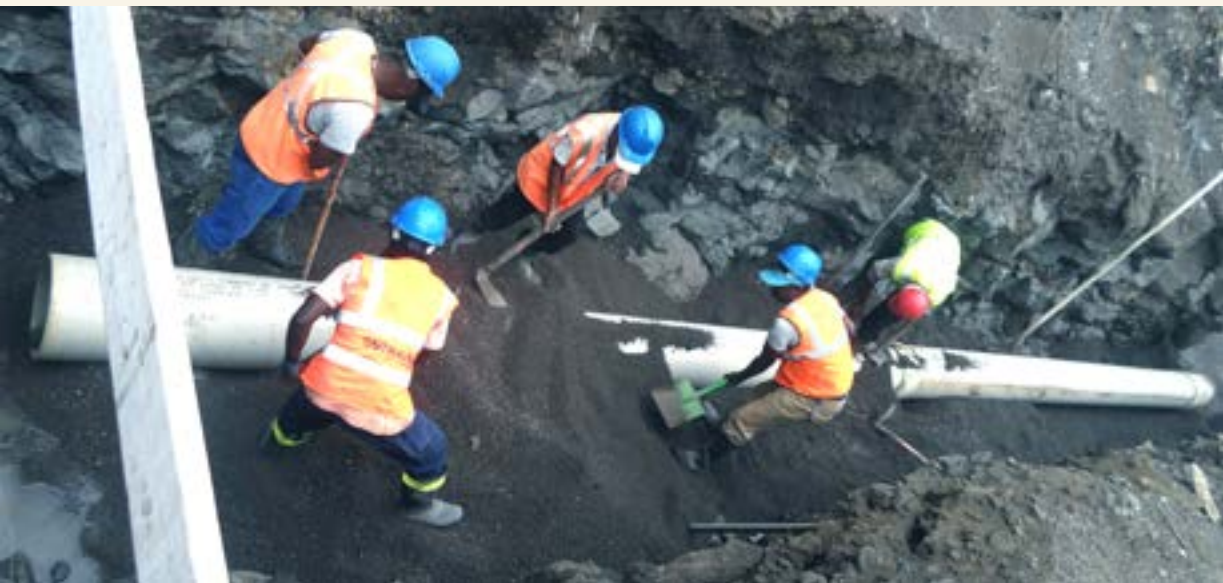
Laying of wastewater pipes
