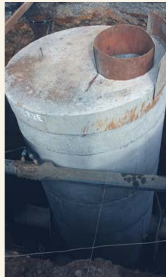
Construction of manhole
