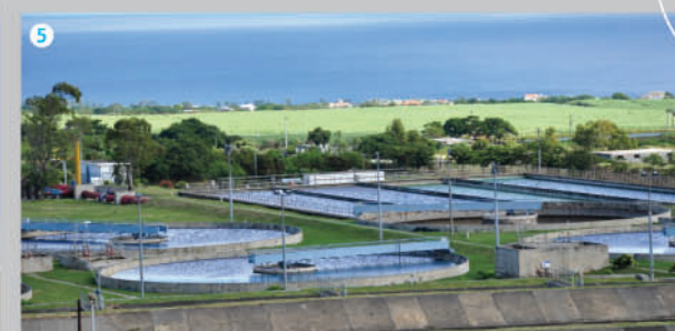
5. The suspended solids with the mixed liquor from the aeration unit is separated from the treated waste by gravity in the final settling tank
