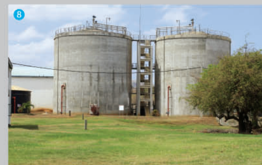
8. The Thickened Sludge undergoes a digestion process in Mesophilic Anaerobic Digesters. The anaerobic digestion reduce the organic material to carbon dioxide, Methane, and other inert end products, in a nutshell biogas production.
