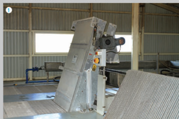
1. The screening system removes all materials up to 6mm, the grit detritor removes sand, gravels, silt, ash and other inorganic materials.
