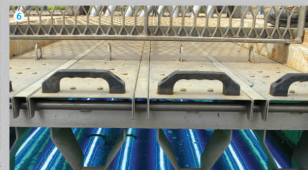
6. Sand filtration and the UV Disinfection: The sand filtration removes any remaining suspended solid from the effluent prior to its disinfection by UV rays.
