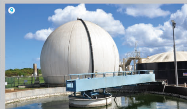
9. The biogas produced also contains hydrogen sulphide which is corrosive to metals and is being used as combustible for the Gas Generator. The present biogas production helps to run the Gas Generator for about 10-12 hrs daily and produces about 25-27% of the plant monthly energy demand.
