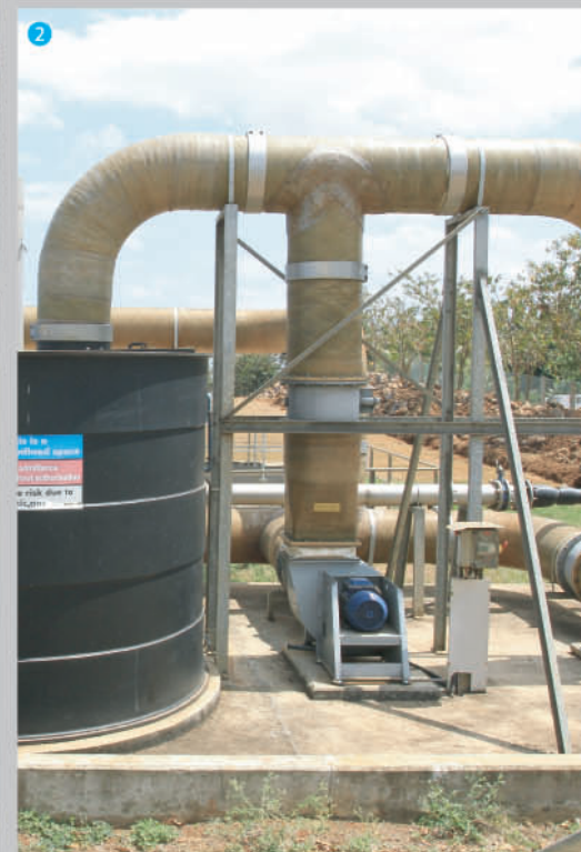
2. Biofilter: The biofilter treats all the air that are extracted from the channel and buildings prior to release to the environment and it is a biological process.
