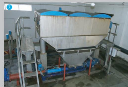
7. The secondary sludge conditioning is effected in a Gravity Drainage Deck with the help of polymers prior to the thickening process.
