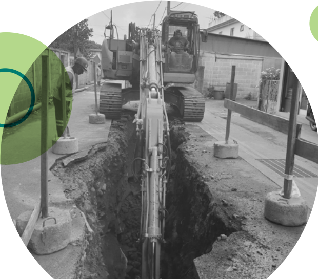
Excavation works for street sewer
