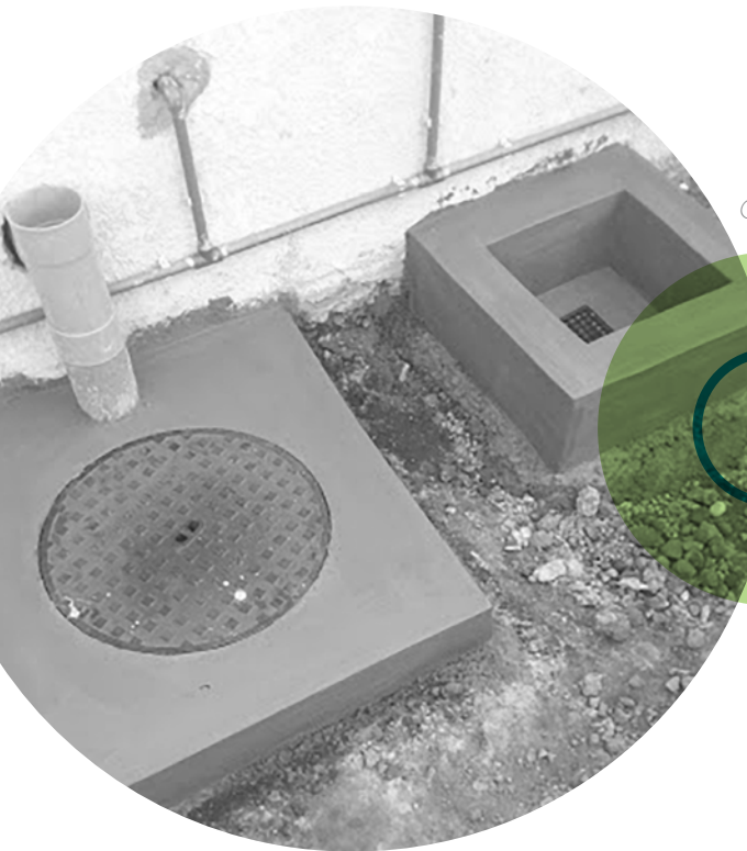
Construction of manhole and gully trap
