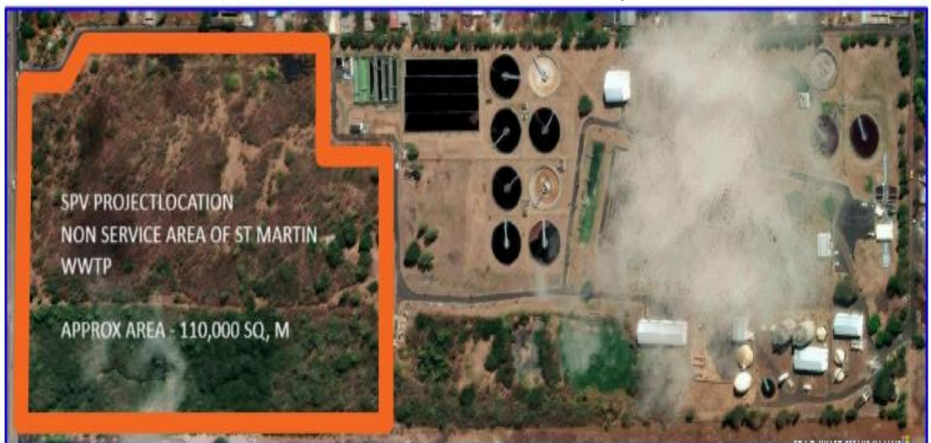
St Martin Wastewater Treatment Plant – SPV Project Location
